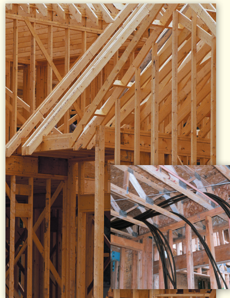
3/4", 1" and 1 1/4" CounterStrike CSST was installed to provide natural gas to each apartment.
